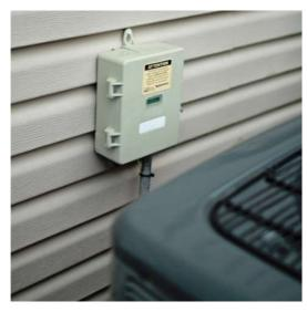
If the customer has a Load Control Receiver (LCR) installed on their home, the compressor on their air conditioner or air-source heat pump will cycle on and off during the event.
