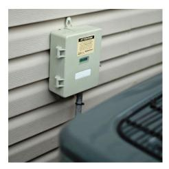
If the customer is participating in SummerSaver with a Load Control Receiver (LCR) installed on their home, the compressor on their air conditioner or air-source heat pump will cycle on and off during the event. MidAmerican notifies customers via email when an event is called.
